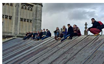
Cohort 2 on top of the roof of Bath Abbey during their core-level training.
