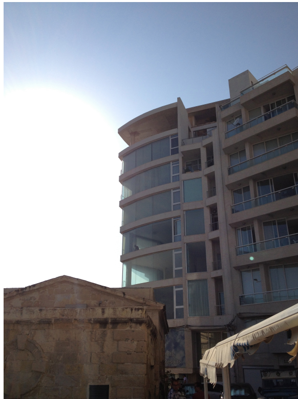
Figure 56: South-East glazed facades of the existing apartment block.
