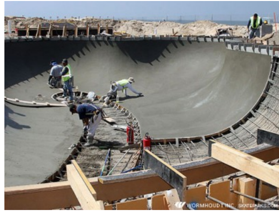
Fig. 153 Construction of the 'Venice Beach Skatepark'.
