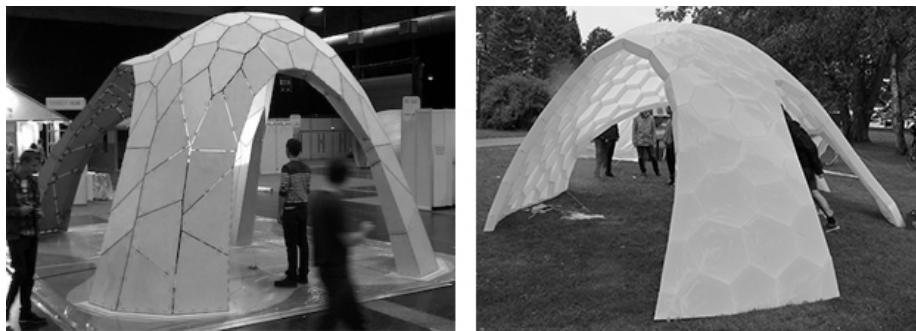
Figure 1.2.1 – Pavilions shaped by dynamic relaxation. Left: Trada Pavilion designed by Ramboll Computational Design. Right: SJ DHL tent designed by Soren Jensen Consultant Engineering
