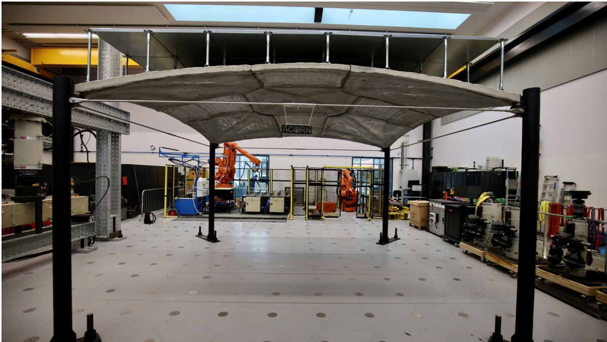
Figure 1: The ACORN concrete shell full-scale prototype [Photo credit : ACORN team at University of Bath, University of Cambridge & University of Dundee]
