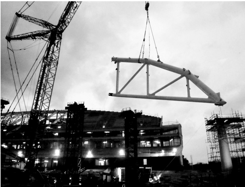
◀ Figure 17: Erection of steel work.
