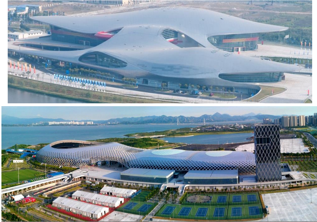
Fig.4 Free-form grid structures with complex boundaries: Guangzhou Sports stadium (above) and Shenzhen Bay Sports Center (below)
