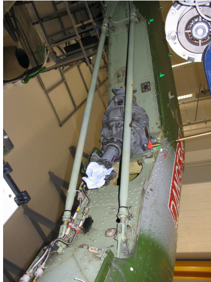
Figure 8.15: Photograph of the 8c struts spanning the corner between the fin and tailboom.
