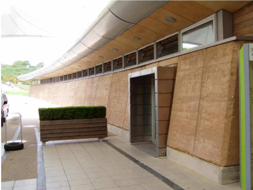
Figure 10.5: Visitors Centre, Eden Project, Cornwall
