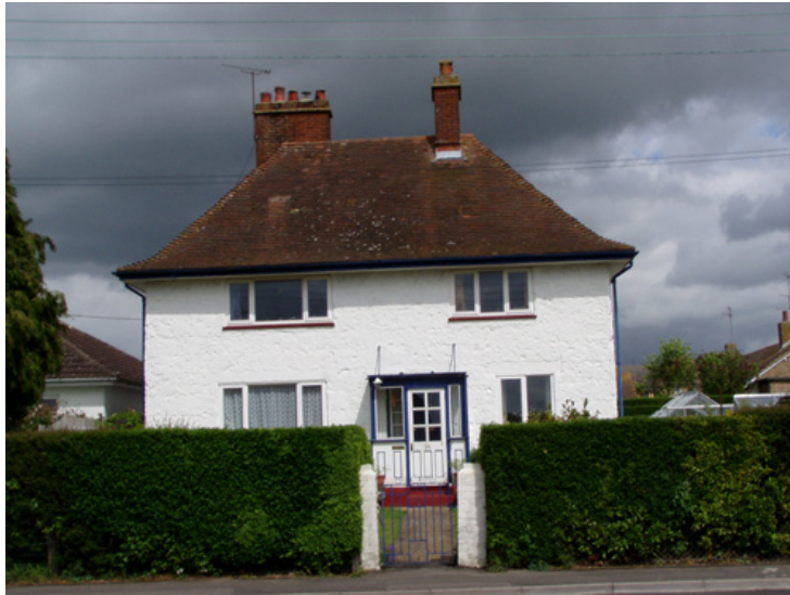
Figure 10.2: Residential rammed chalk property in Amesbury, Wiltshire
