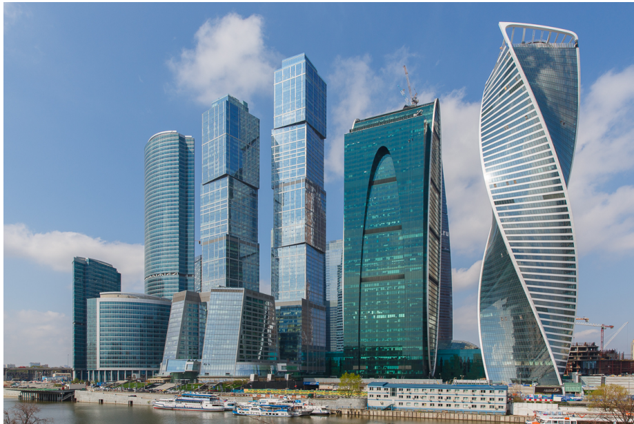
Figure 1: Examples of glazed, unitized curtain walls enclosing buildings at the Moscow International Business Center.
