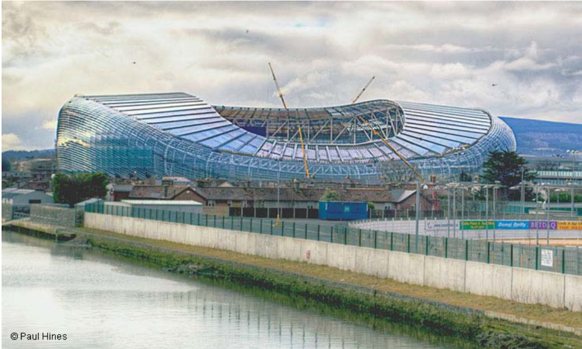
Fig. 1 New stadium near completion
