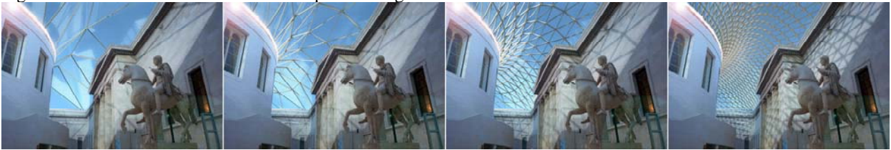
Fig. 3 British Museum Great Court roof options using various levels of subdivision
