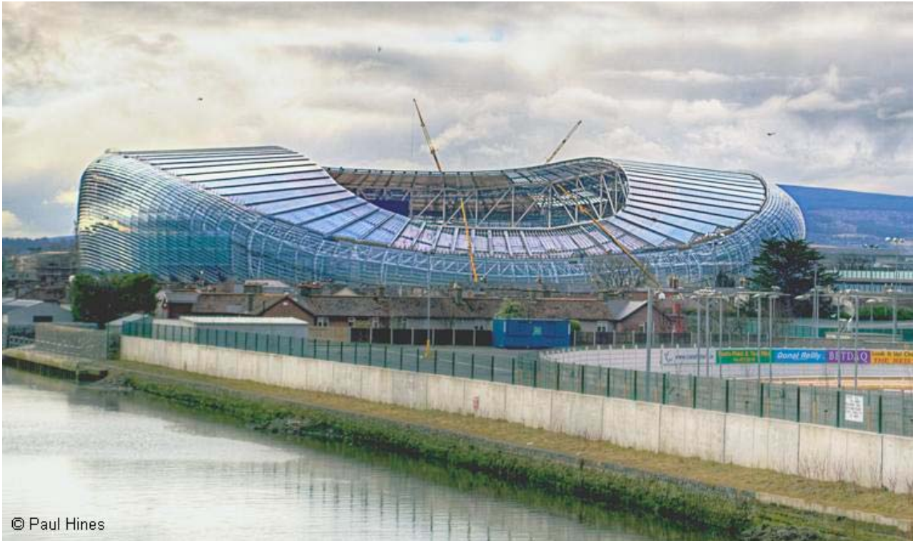
Fig. 4: Aviva Stadium near to completion
