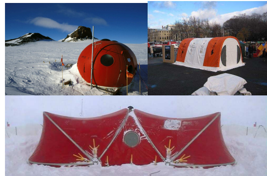
Fig. 8: Structures with different curvature: a rigid module with synclastic shape from Wallhead (top left); a fabric shelter from a developable surface, Weatherheaven (top right) and the Stratuggi Room from a set of anticlastic surfaces, ARQZE (bottom).
