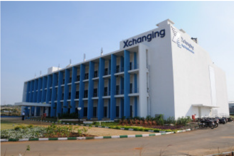
Figure 10: Completed Xchanging building upon which this study was based
