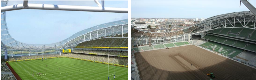
Figure 2: Aviva Stadium roof - computer render (left) and photo (right)
