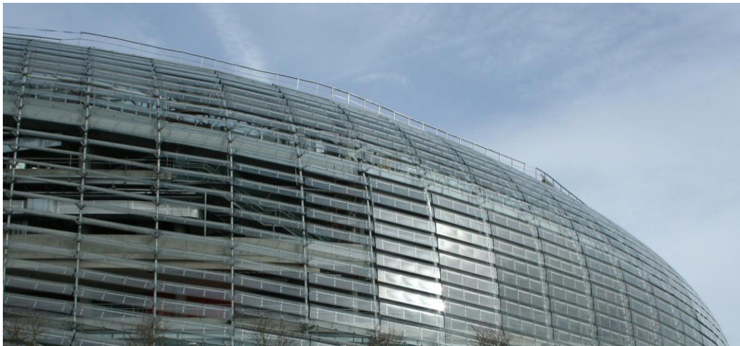
Figure 3: Aviva Stadium louvres transition from open (left) to closed (right).
