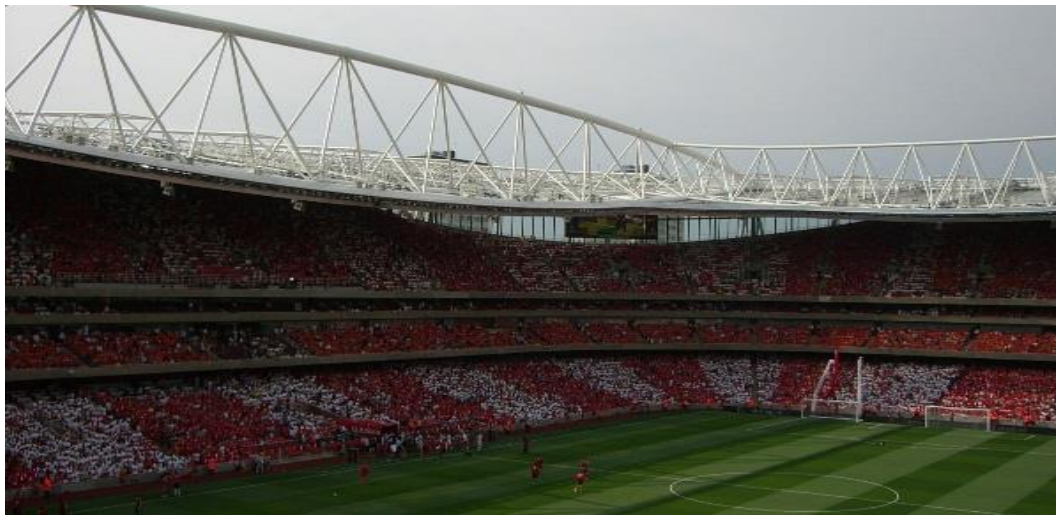
Figure 6: Emirates Stadium roof truss
