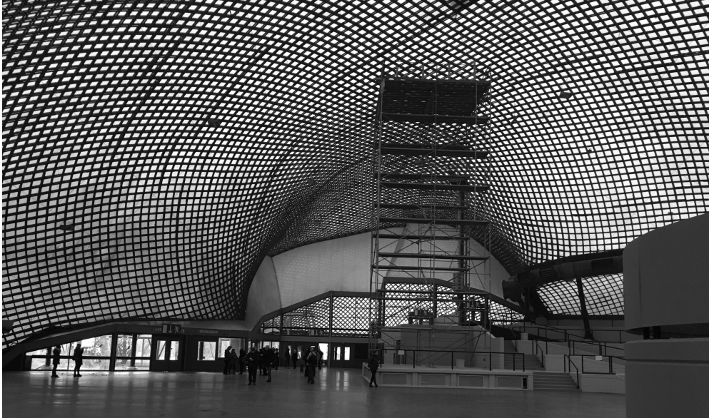
Figure 1: Mannheim Multihalle, Germany 1974. Frei Otto, Carlfried Mutschler and Winfried Langner, Ove Arup and Partners
