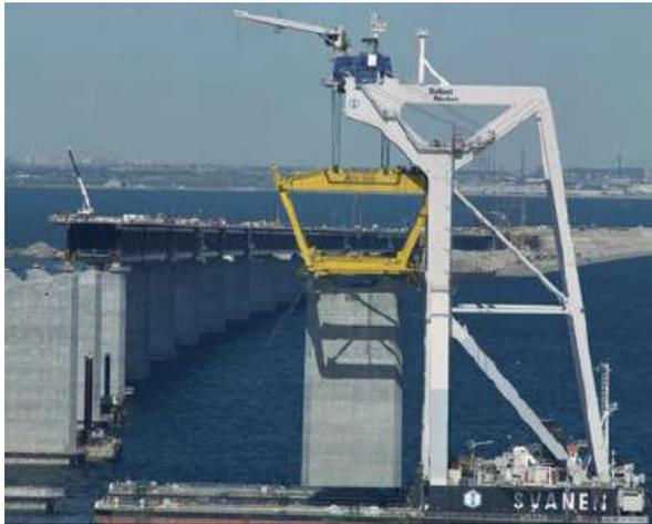
**Figure 6:** “Svanen” used for the construction of the Oresund Bridge
