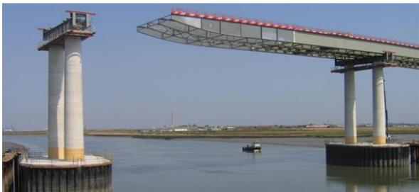
**Figure 7:** Launching of the deck using a steel nose across the central span of the bridge
