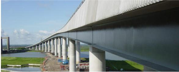
**Figure 4:** View of fascia and parapet
