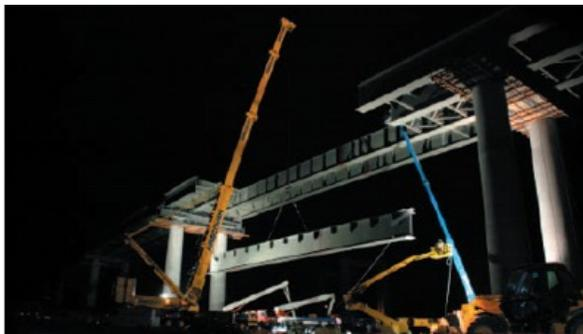
**Figure 10:** Lifting of deck girders into place
