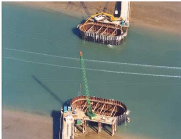
**Figure 12:** Construction of cofferdams via temporary jetties
